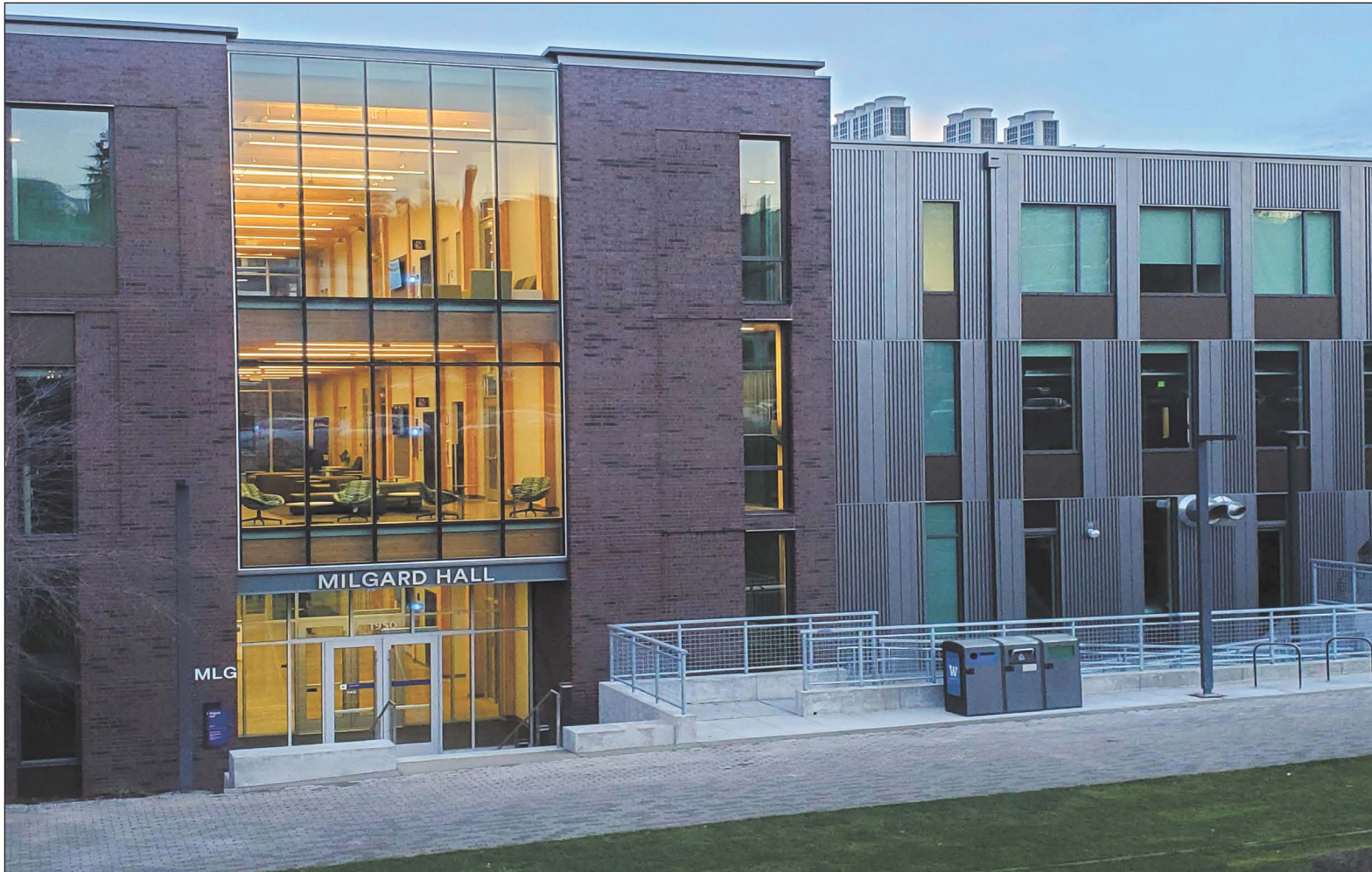
Milgard Hall before demolition slated for April 31.
